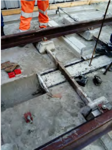
< Coffrage cunette diam 360 mm
